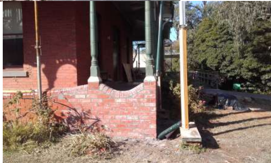
New brickwork — nearly finished!
